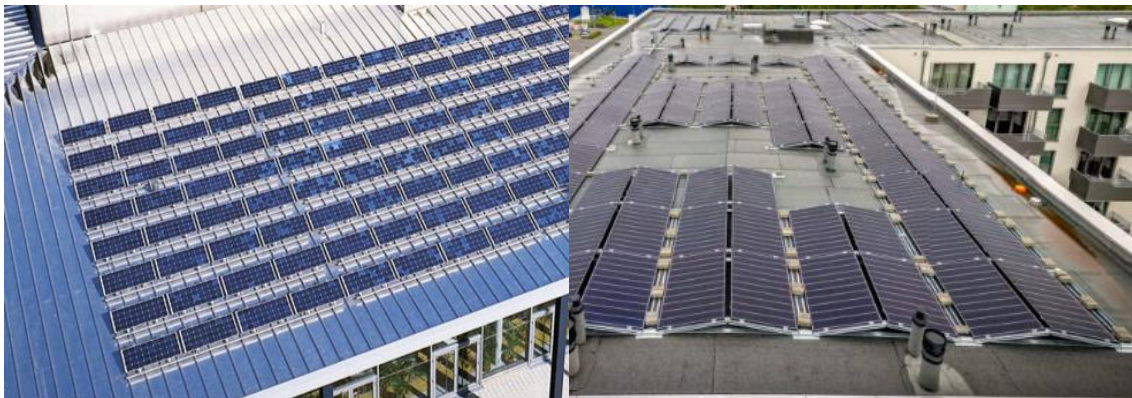
Figure 3: South oriented module rows (left) in comparison with alternating east-west-oriented module rows (right).
